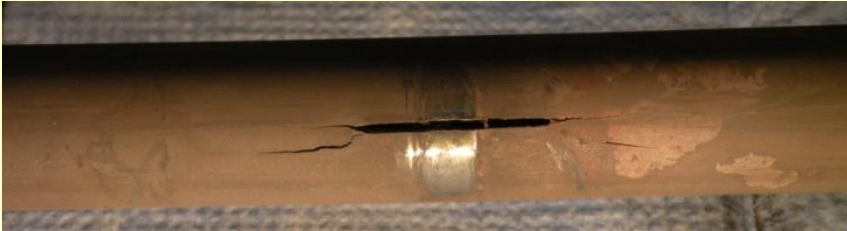
Cracked pressurizer heater
