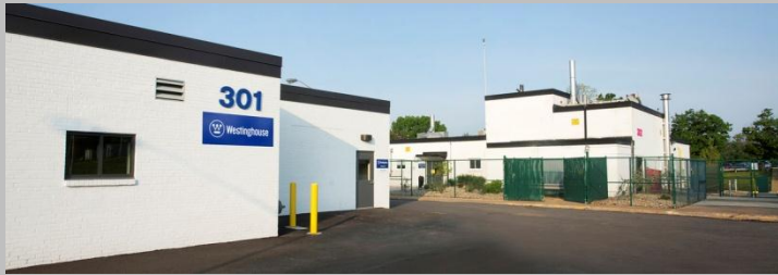
Westinghouse Materials Center of Excellence Laboratories and Hot Cell Facility, Churchill, Pennsylvania (USA)
